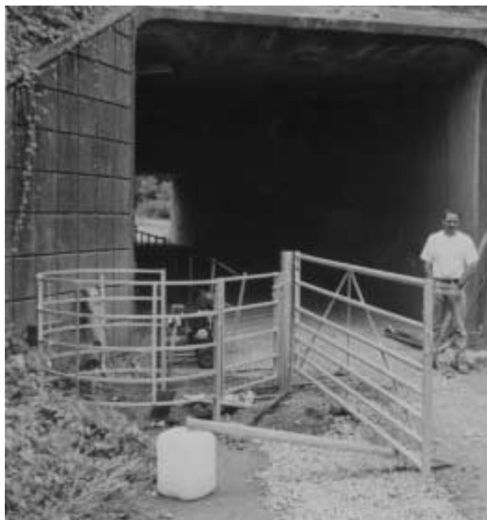
Contractors install barriers at Strood underpass.
