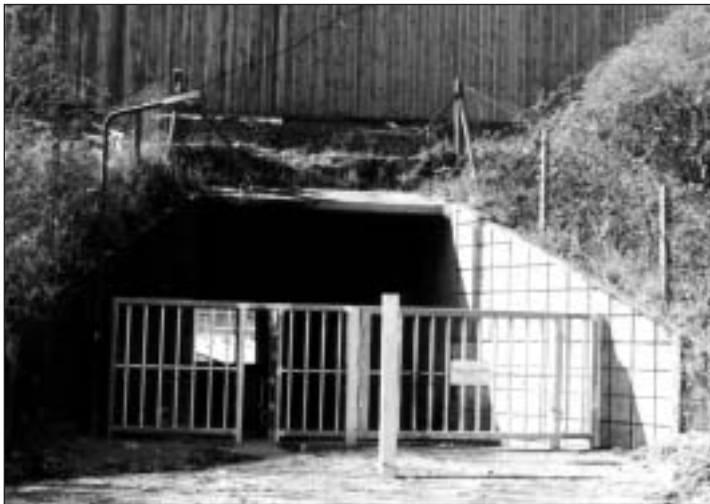
The new barrier at Temple Wood underpass
