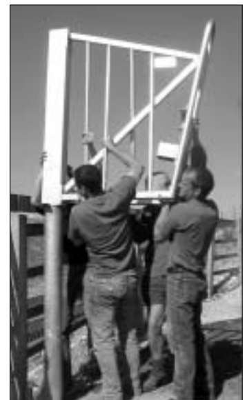
The new gate near Merrals Shaw
