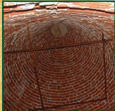
Interior of the brickwork cone
