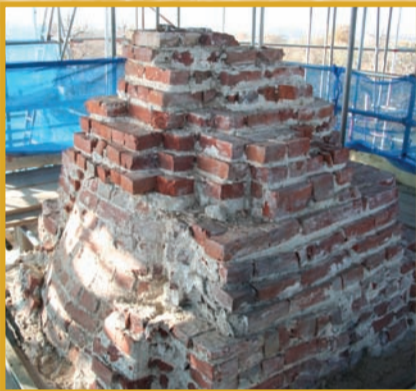
Top of the brickwork cone
